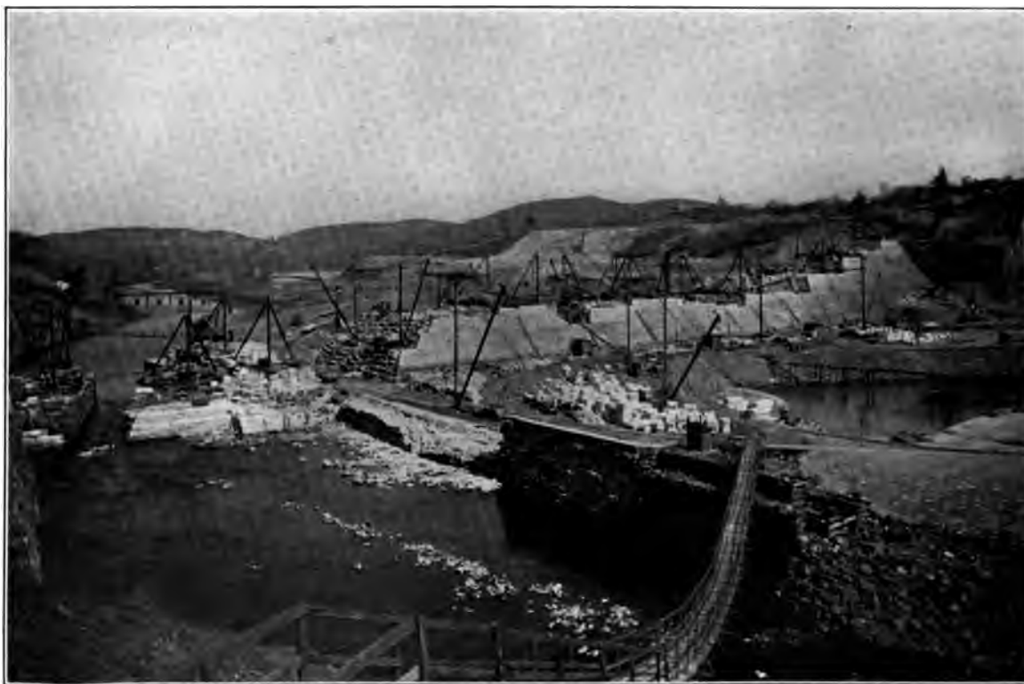
NEW CROTON DAM. LAYING MASONRY ACROSS TEMPORARY CHANNEL.
