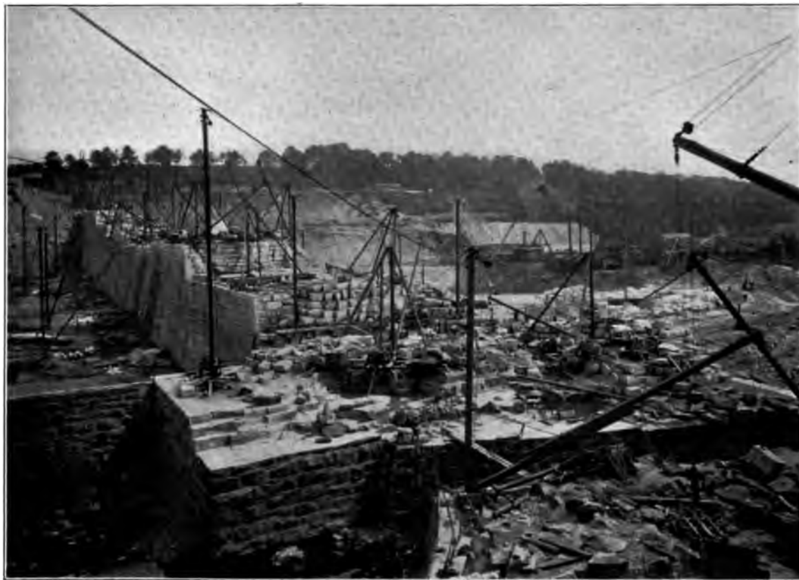
NEW CROTON DAM. UP-STREAM FACE.
