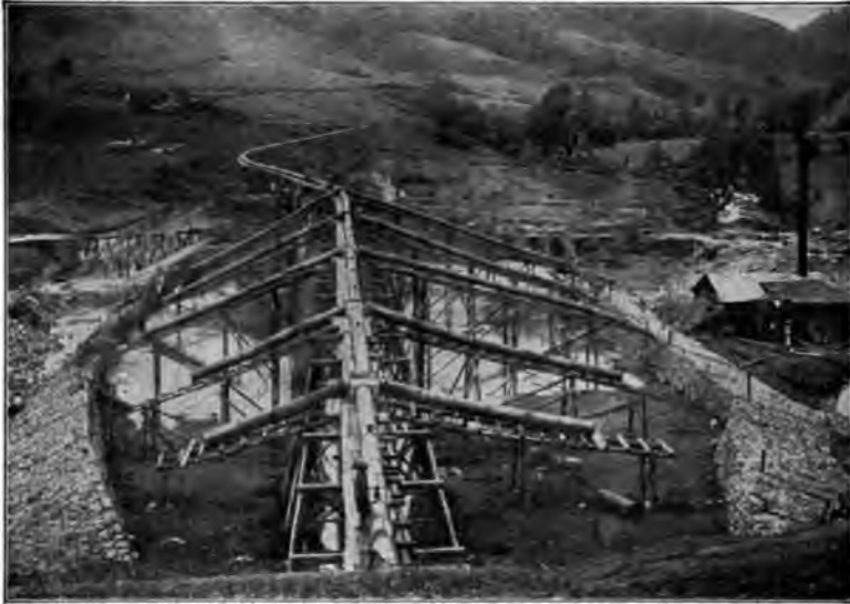
FIG. 59.—DAM NO. 1, TENANGO RIVER. Distributing Sluiced Materials through Pipes.
