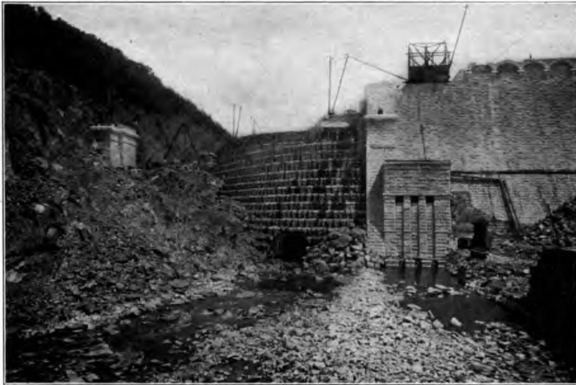
NEW CROTON DAM. RELIEF OPENINGS IN DAM.
