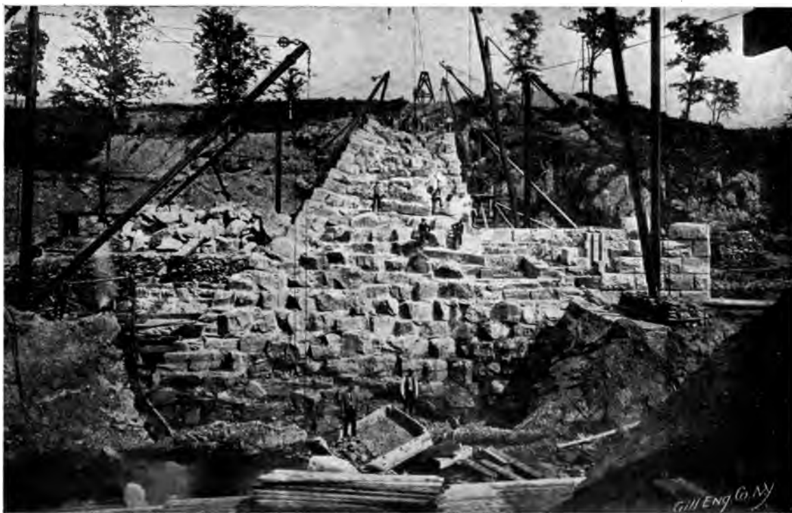
SODOM DAM, IN CONSTRUCTION.
