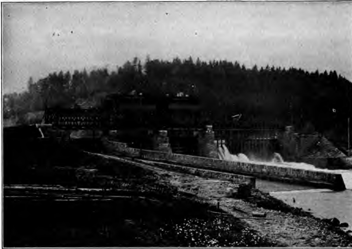
DAM FOR HYDRO-ELECTRIC PLANT AT HAGNECK, SWITZERLAND.
