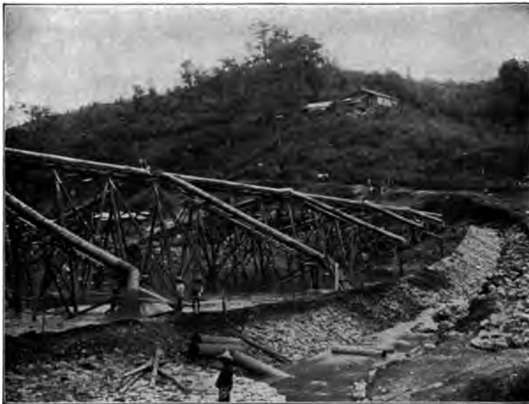
FIG. 60.—DAM NO. 1, TENANGO RIVER. Depositing Liquid Earth through Pipes on Down-stream Slope.
