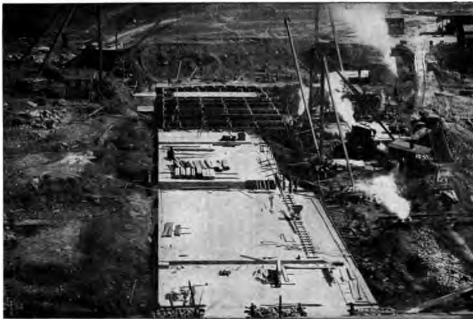
JUNIATA DAM. FLOOR NEARLY COMPLETED.
