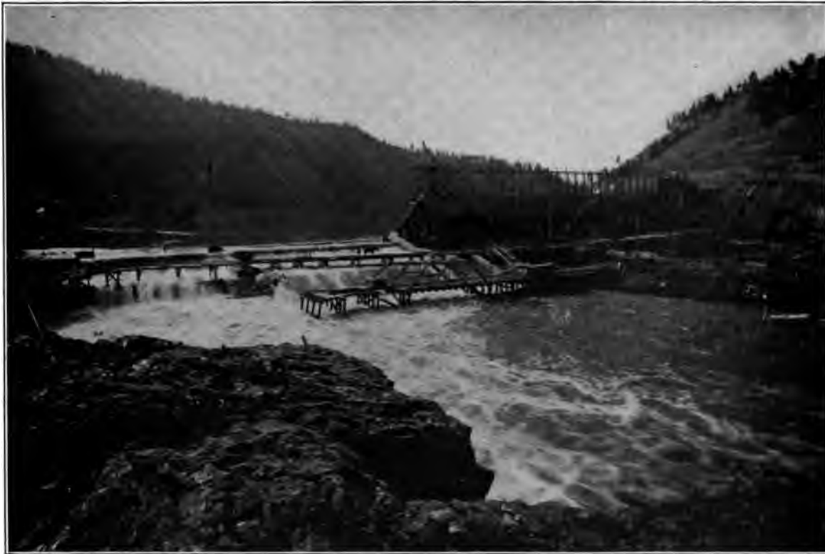
HAUSER LAKE DAM IN CONSTRUCTION.
