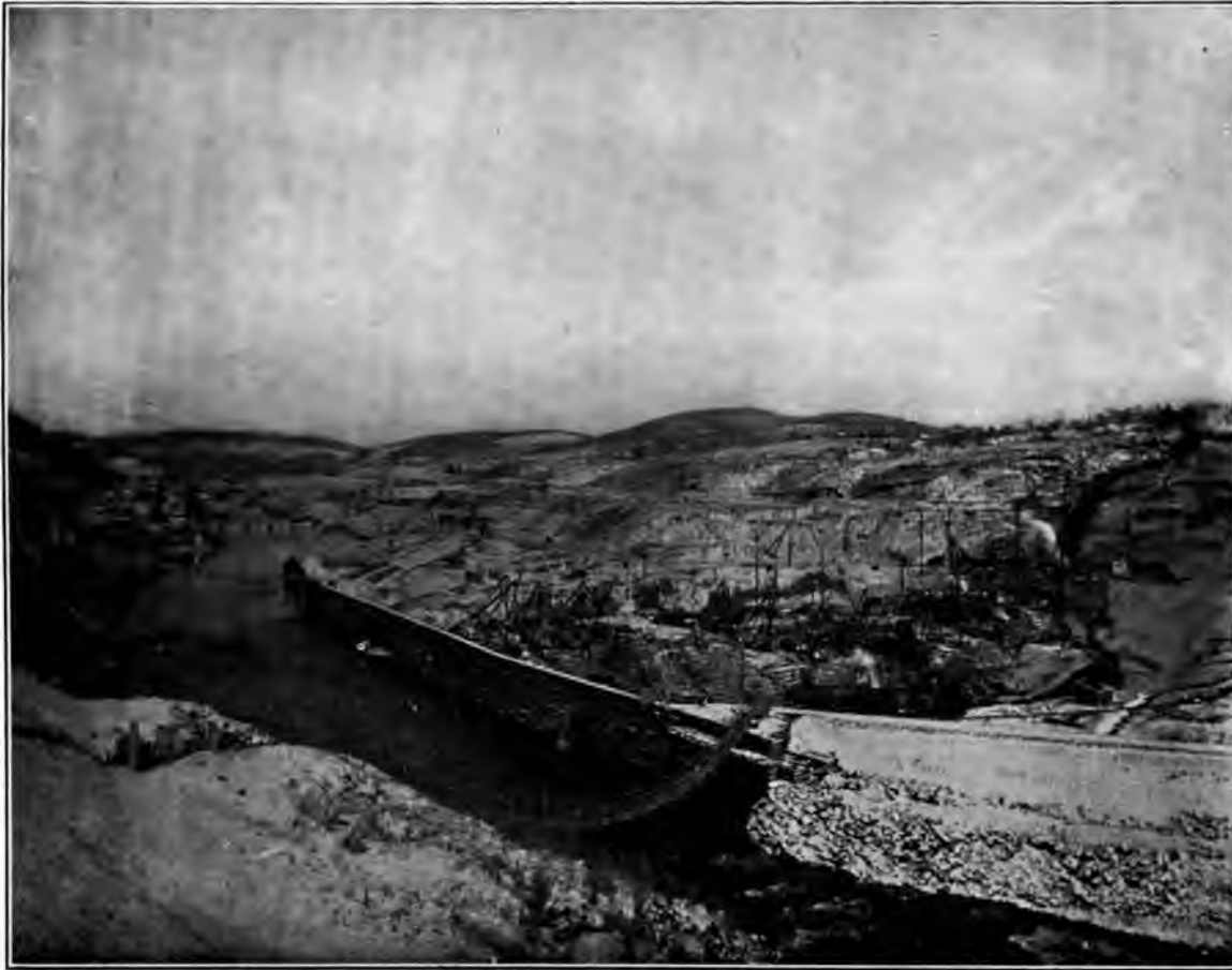
NEW CROTON DAM. TEMPORARY CHANNEL.
