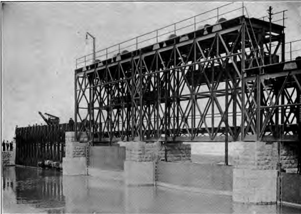
DAM FOR HYDRO-ELECTRIC PLANT AT HAGNECK, SWITZERLAND, SHOWING STONEY SLUICE-GATES.
