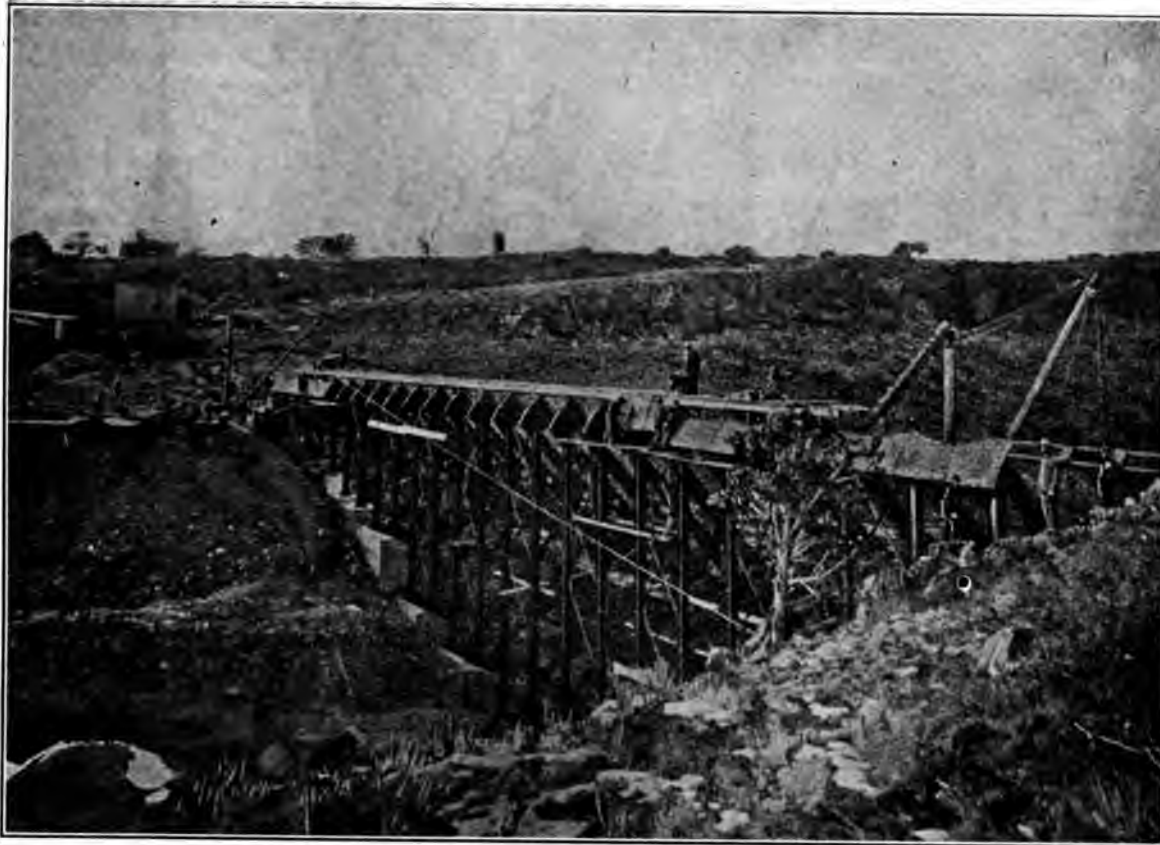
ASH FORK STEEL DAM.
