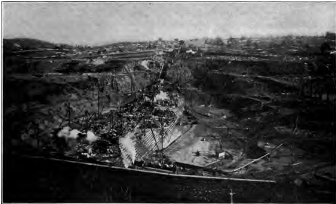
NEW CROTON DAM. LAYING MASONRY IN FOUNDATION TRENCH.
