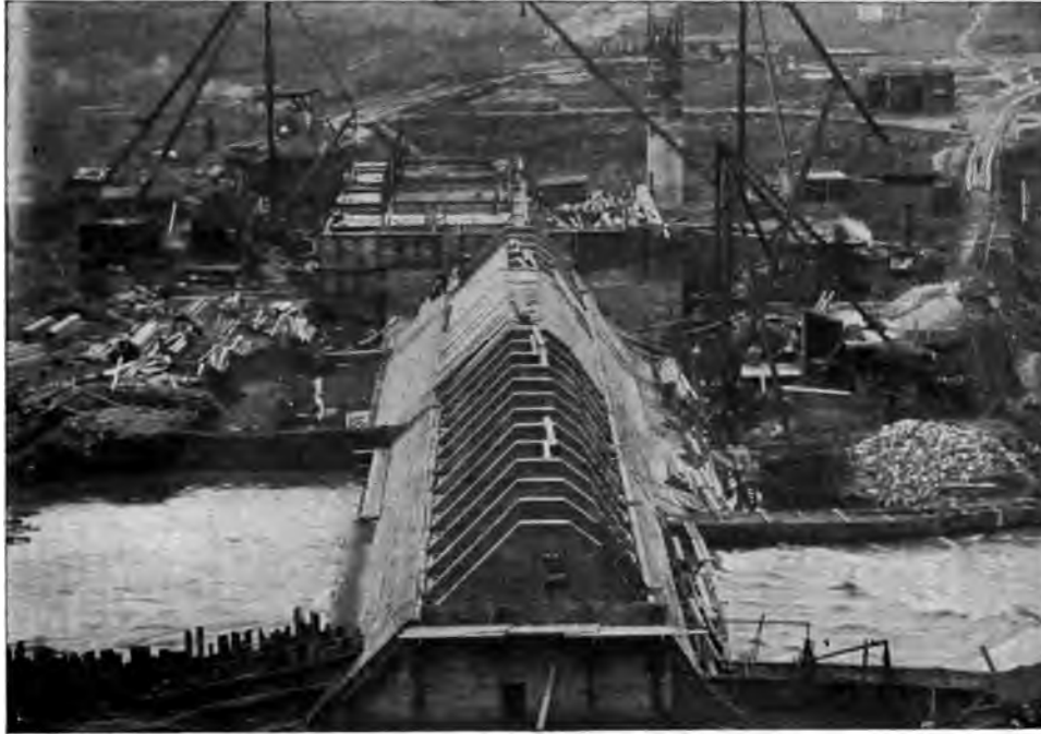
JUNIATA DAM. SHOWING CONSTRUCTION OF BUTTRESSES AND DECK.
