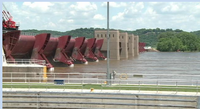
Lock and Dam 11 in Dubuque
