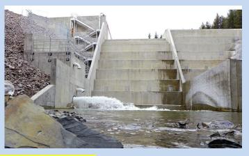
concrete structure that six years ago was deemed inadequate. At the time, Morrison-Maierle completed a core sample test of the arch dam and found its concrete strength was less than 1,000 pounds per square inch. Normal strength is between 3,000 and 4,000 pounds per square inch.
