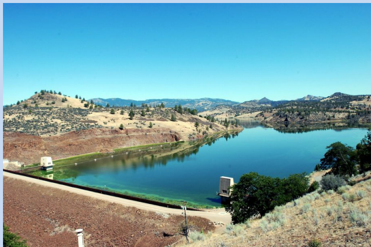
Iron Gate Dam on the Klamath River near Hornbrook (Siskiyou County), seen in 2009, is one of the dams set to be taken down in a river restoration project. Less Iron Gate Dam on the Klamath River near Hornbrook (Siskiyou County), seen in 2009, is one of the dams set to be taken down in a river restoration project.
