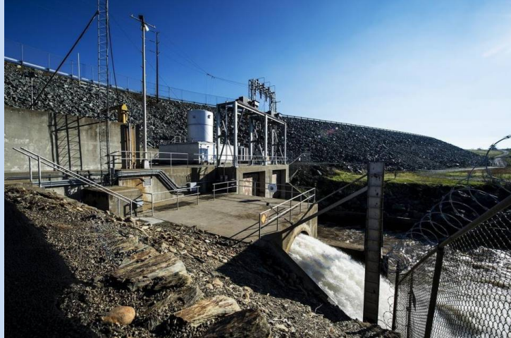
Water flows through the McSwain Dam in Snelling on Wednesday, Dec. 30, 2015. According to Bill Cochran, project manager of the Merced Irrigation District's New Exchequer Hydroelectric Project, the McSwain powerhouse is capable of producing 10 megawatts of power. Andrew Kuhn akuhn@mercedsunstar.com
