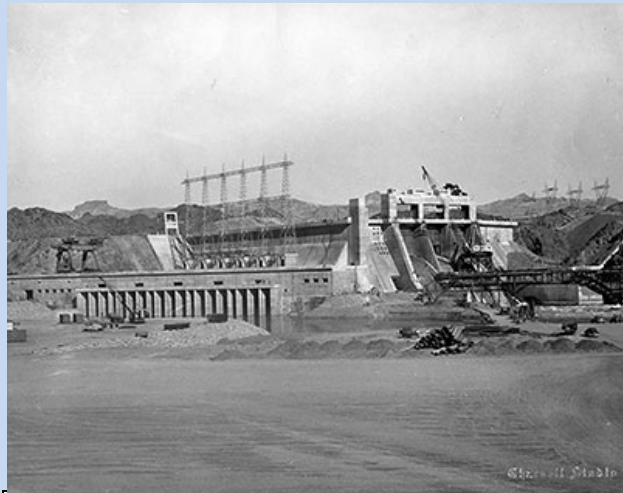
Courtesy - Work continues on Davis Dam in 1946.
