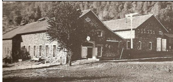
Volta Powerhouse at Manton built in 1901; demolished by PG&E in the 1980s
