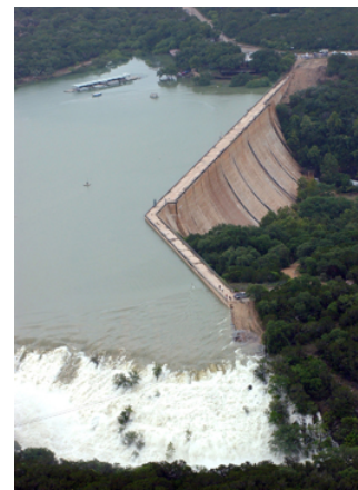
Note: Water flowing around right abutment during flood
