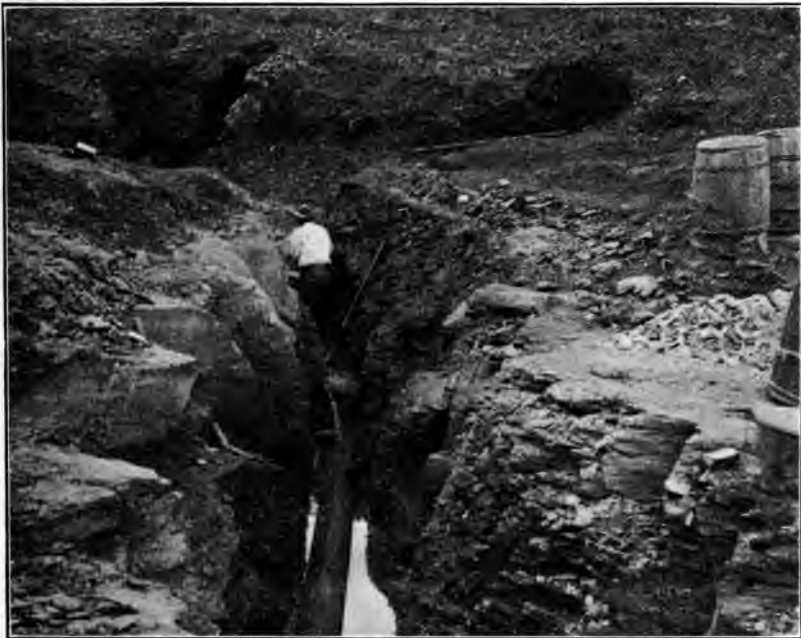
FIG. 9.—VIEW OF MAIN CENTRAL DRAIN, TABEAUD DAM.
