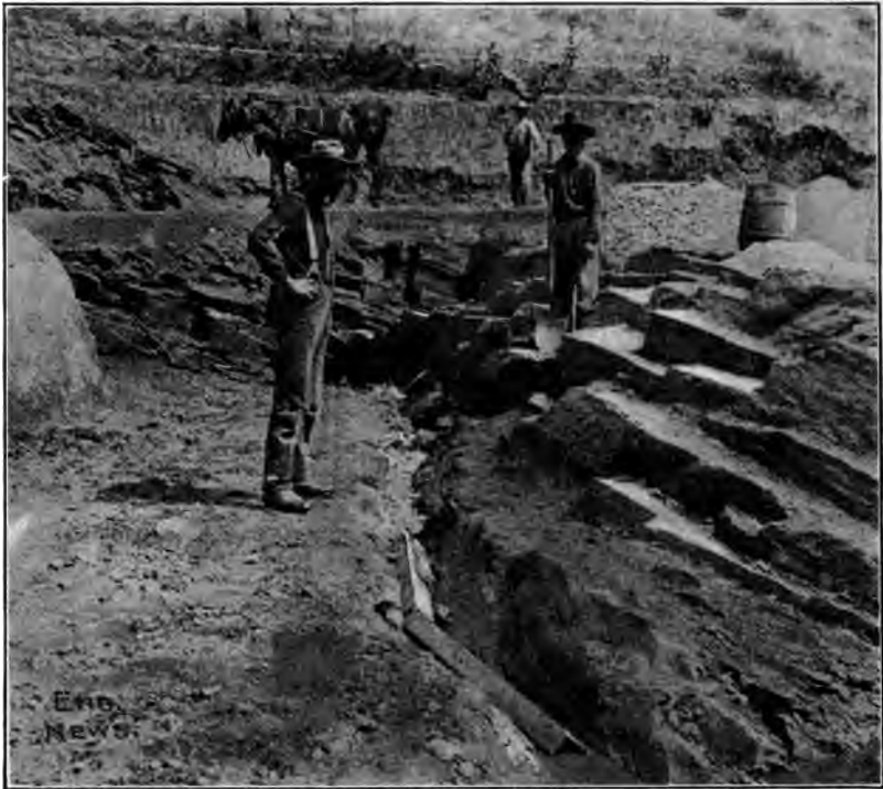
FIG. 7.—VIEW OF NORTH TRENCH, TABEAUD DAM.
