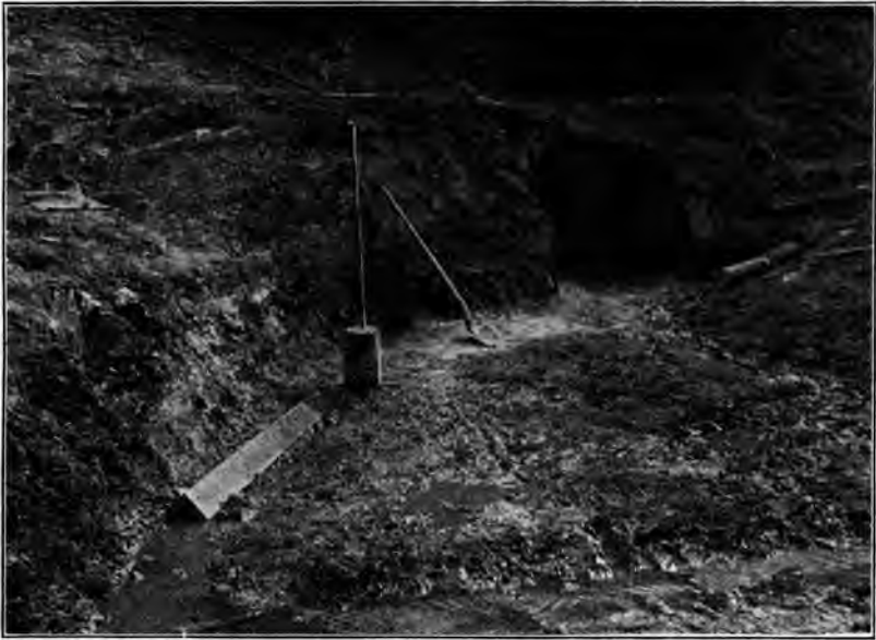
FIG. 8.—VIEW OF SOUTH TRENCH, TABEAUD DAM.
