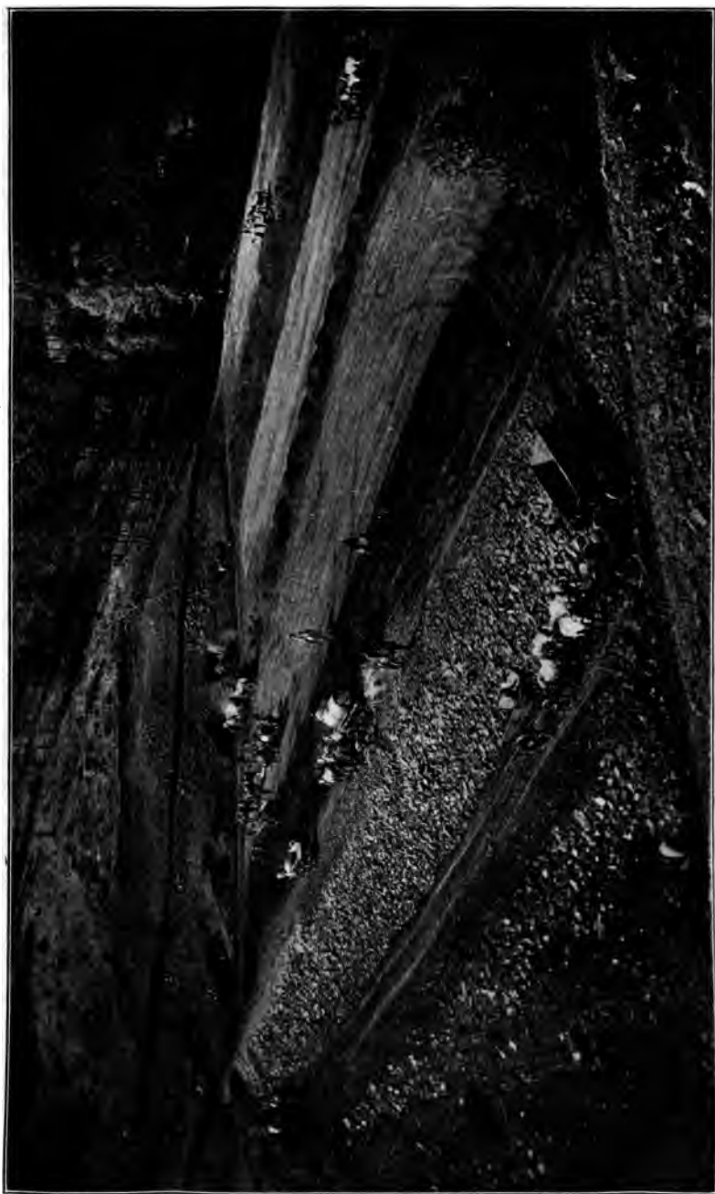
FIG. 10—VIEW OF TABEAUD DAM WHEN ABOUT HALF COMPLETED.
