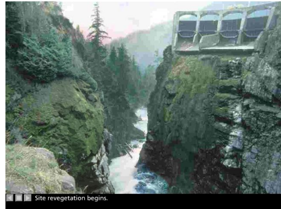
Glines Canyon Dam Removal Process
