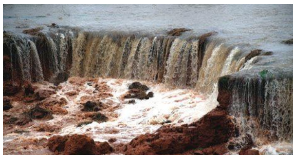
The emergency spillway at the Golf Course of Oklahoma continues to erode away beneath the powerful flow of flood waters.
