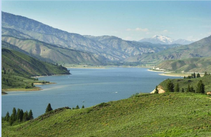
Anderson Ranch Reservoir east of Mountain Home stores water on the South Fork of the Boise River. The Cat Creek Energy hydro project would draw water from the lake into a new reservoir at a higher elevation and then run it through turbines to produce energy as it returns to Anderson Ranch. Idaho Statesman file
