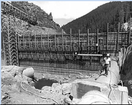
Construction of Stagecoach dam in August 1988.
