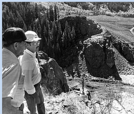
Construction of Stagecoach dam in September 1987.
