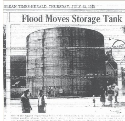
In 1942, rainfall in Smethport, Pennsylvania was estimated to be nearly 31 inches in less than 5 hours. This estimate exceeds the hypothetical PMP. The flood waters picked up and moved this water tank well downstream.
