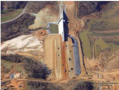
Aerial view of zoned earth embankment construction
