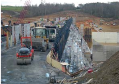
Typical RCC placement
