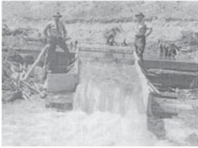
Modeling of hydraulic structures has been performed since the 1800s. This model was undertaken in 1936 for the design of Poe Dam in Pennsylvania.
