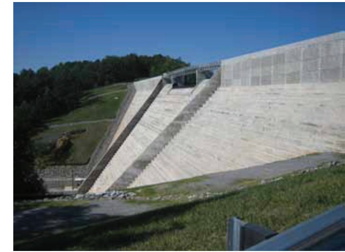
Hickory Log Dam, Canton, Georgia
