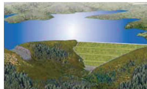
New Ragged Mountain Dam Charlottesville, Virginia
