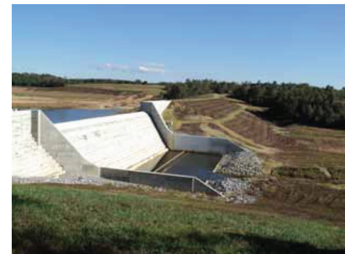
Deep Creek Dam 5D, Yadkin County, North Carolina
