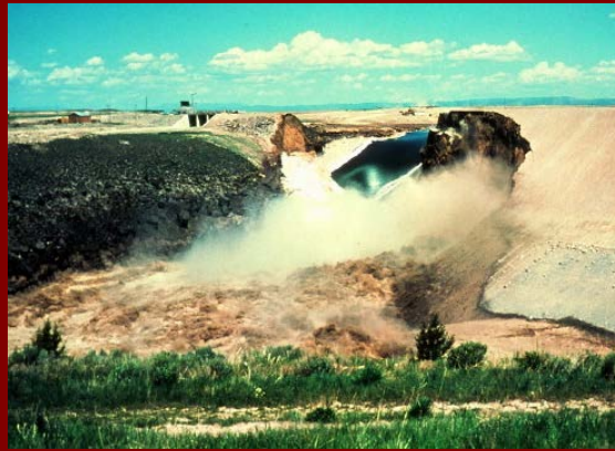
Teton Dam Failure on First Filling
