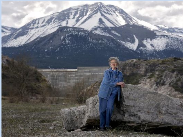
Eloise Erickson stands next to a rock slab that was part of the original 1912 Swift Dam which failed on June 8, 1964. Boulders weighing as much as 80-tons were pushed more than half a mile when the dam collapsed. The current Swift Dam is a 205-foot high concrete dam that was completed in 1967.
