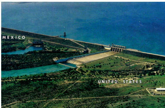
Falcon Dam and Reservoir. This international dam creates a reservoir of some 3,978,416 acre-feet for flood control, conservation and hydroelectric generation as well as recreational uses. The international boundary crosses the center of the dam.
