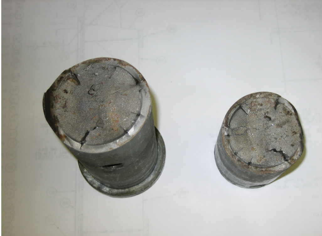
Photo 3: Wanapum Dam, Tainter Gate 1, left bank hoist chain, roller pin 41 end view
