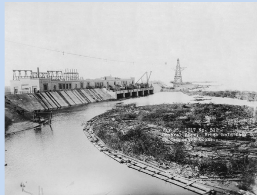
Lake Wissota Dam construction in 1917 (Image: Chippewa County Historical Society)
