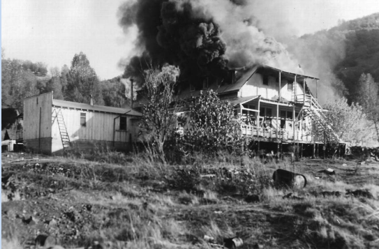
The Bidwell Bar store was burned, along with the rest of the town, in 1964 to make way for the inundation of the area by Lake Oroville. Courtesy of Larry R. Matthews
