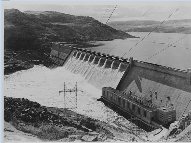
Grand Coulee Dam on the Columbia river, Washington (Farm Security Administration - Office of War Information Photograph Collection (Library of Congress))
