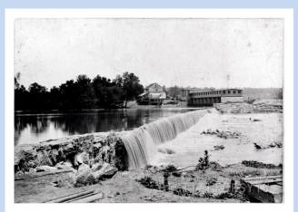
began in 1897 and it soon became known as Idol's Hydroelectric Station, after a ferry that was once located on the same site. The dam built for the station was 482 feet long and the reservoir covered about 35 acres. The flow of the dam generated about 2,500 horsepower. The station later provided power for other textile and grain mills, fertilizer plants, the Winston-Salem electric railway, electric street lights and wood and metal working shops in Winston-Salem.
