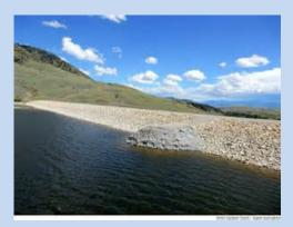
Its crest also has moved about 8 inches downstream. The district already has spent about \$1.5 million to install instruments to measure the dam's movement. It has considered possible repairs ranging from injecting concrete into the dam to shore it up to rebuilding it. The latter is something
