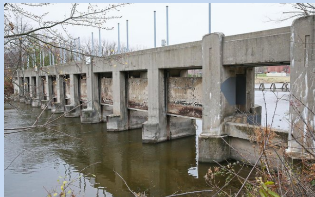
Milwaukee County officials set a late June start for repairing the deteriorated Estabrook Park dam on the Milwaukee River and building a fish passage around its north end at a cost of $3.4 million, in a revised schedule given to the state Department of Natural Resources. The four gates on the right would be removed for construction of a fish passage.
