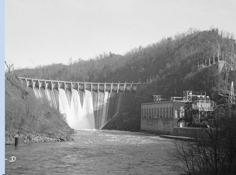
The Cheoah Dam, built by Alcoa in 1919, photographed by the Tennessee Valley Authority in 1939. (Photo: Courtesy photo)
