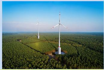
base of each tower is a water reservoir containing 1.6 million gallons of water. The four towers are daisy chained by a channel that takes water down a valley to a 16-megawatt pump/generator hydropower plant. The site will house another reservoir holding 9 million gallons of water for additional water storage.
